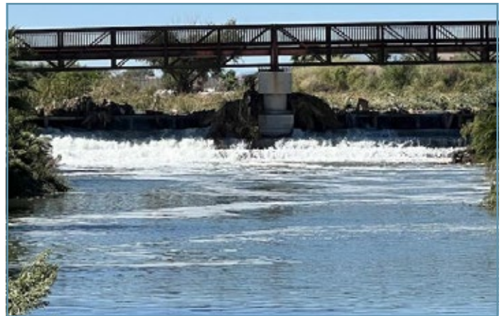
Bridge in Wetlands Park over Las Vegas Wash
